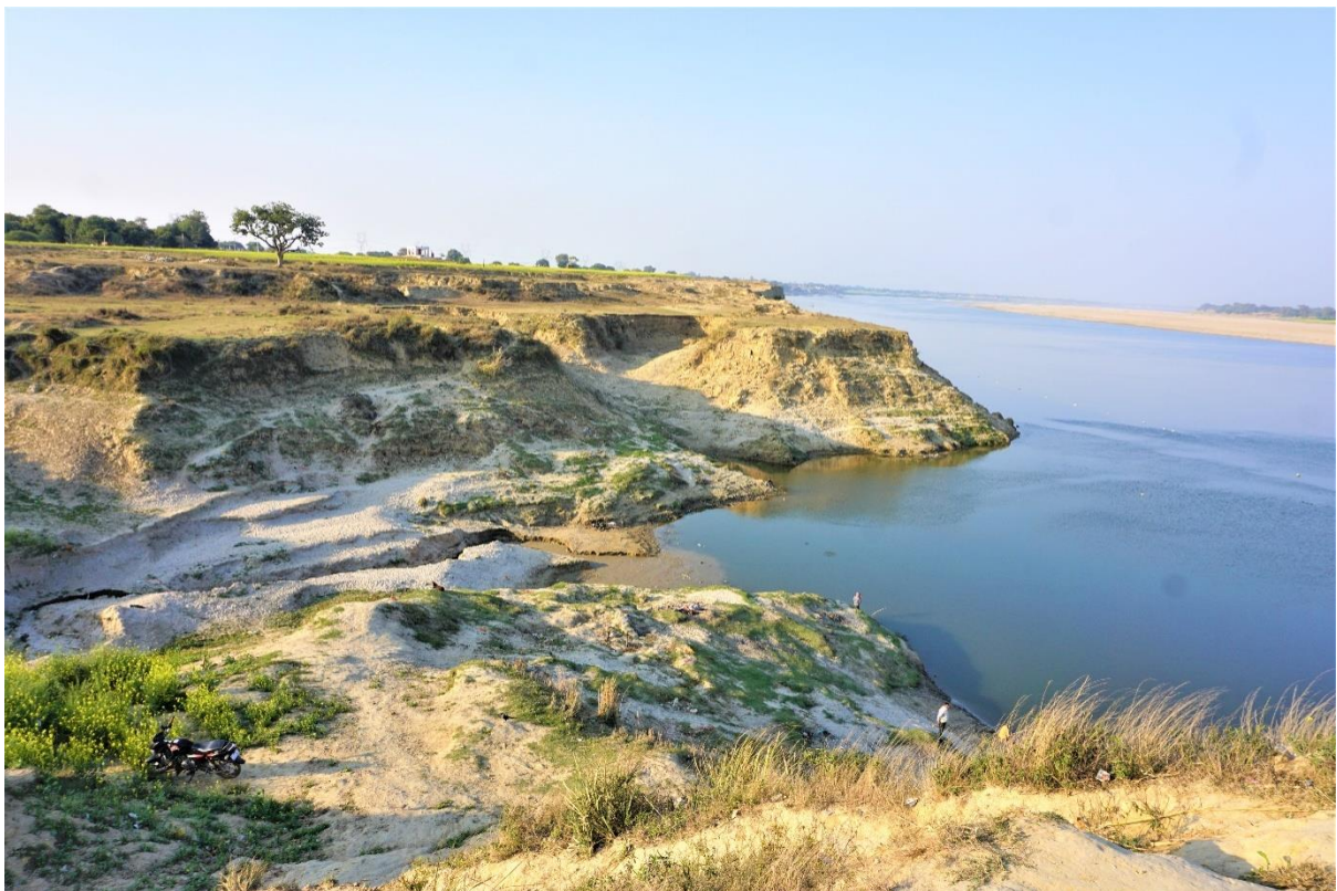
Image 65 : Eroded Bank Near Birukhar Village [Right bank]
