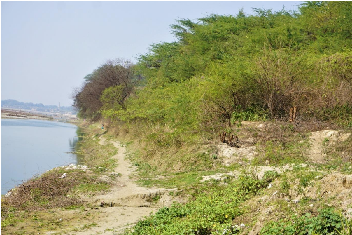
Image 58 : Stable Bank of River Ganga Between Ramchaura And Sringerpur [left Bank]
