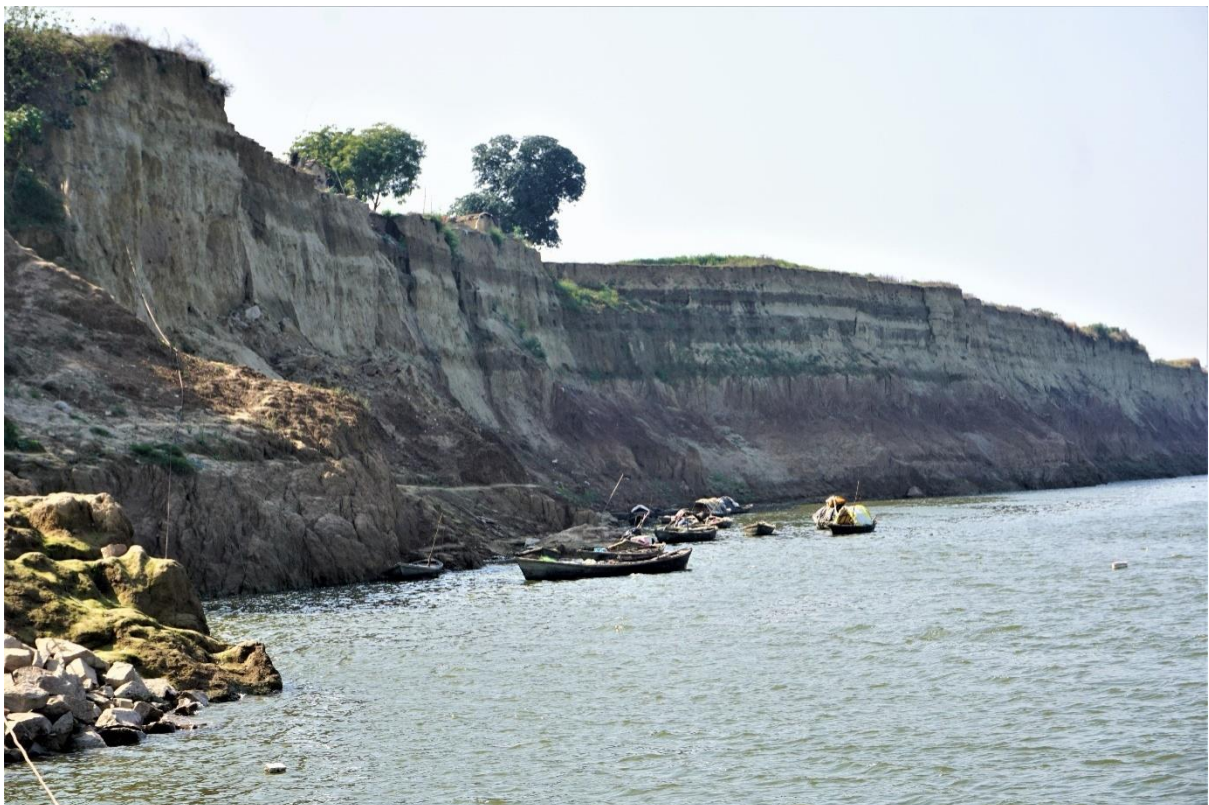
Image 63 : Erosion Prone Bank In Kusamha Village [Right Bank]
